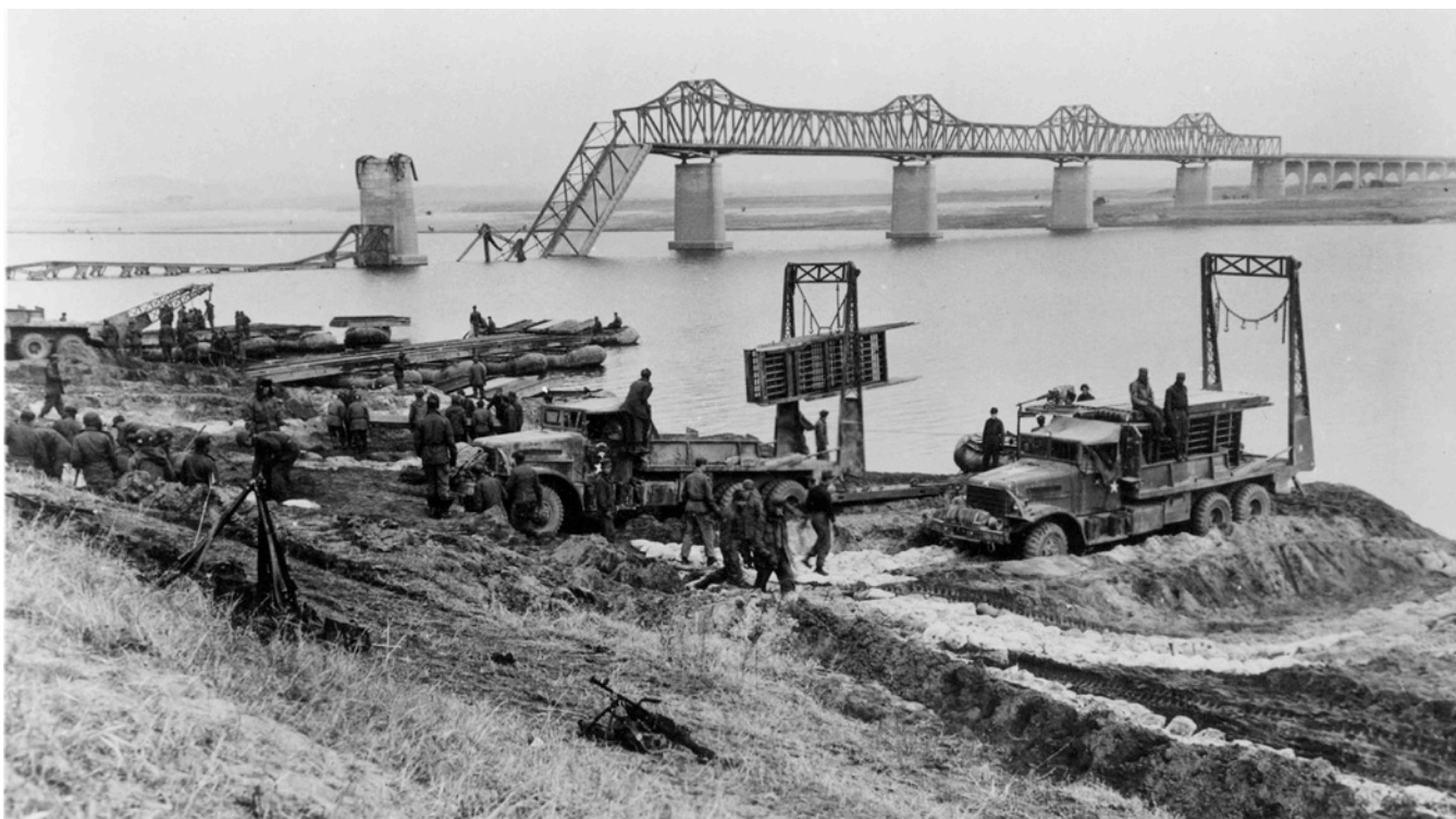
December 9, 1950, Members of the 55 th Engineer Treadway Bridge Battalion, I Corps, construct a floating bridge across the Han-gang. The western most railroad bridge is seen in the background. (U.S. Army, Courtesy of Harry S. Truman Library)
